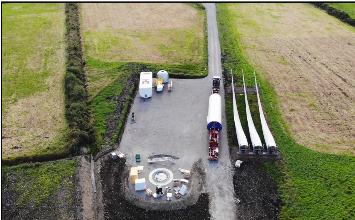
Figure 4.9 Typical finished hardstand on a wind farm
