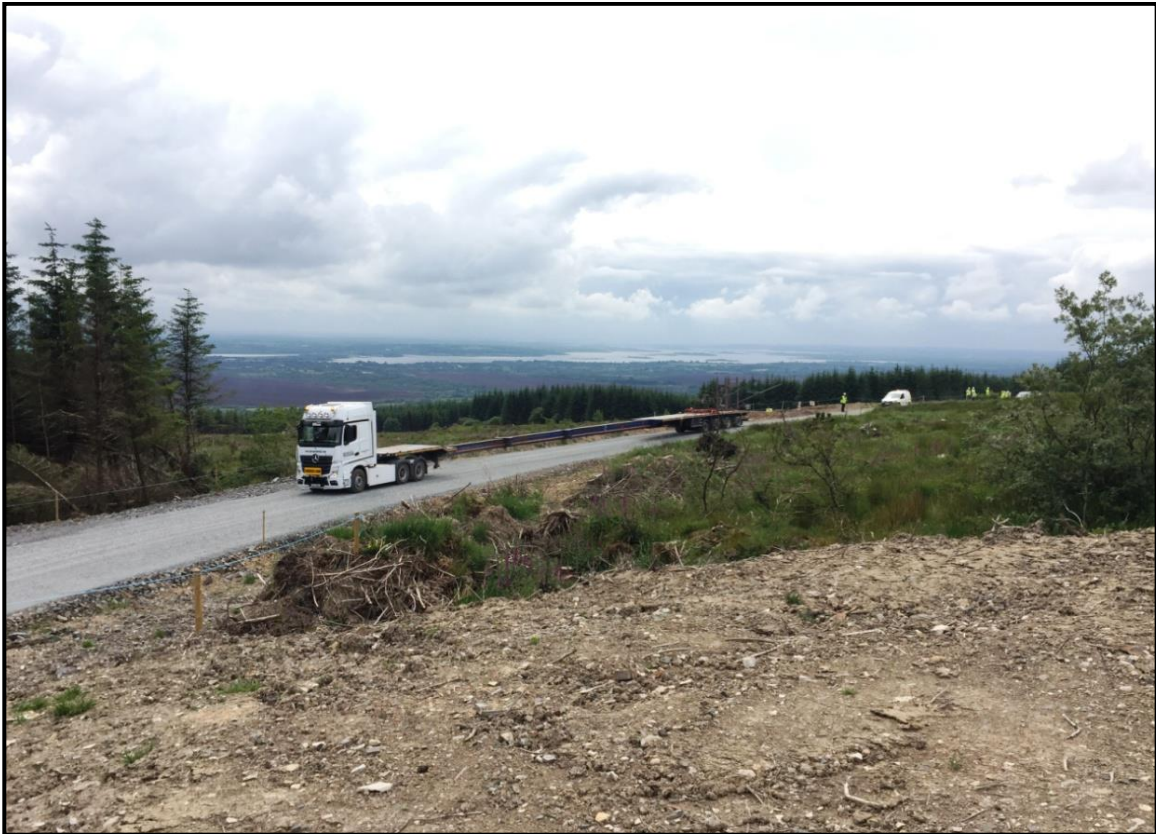
Figure 4.2 Typical upgraded forestry road on a wind farm
