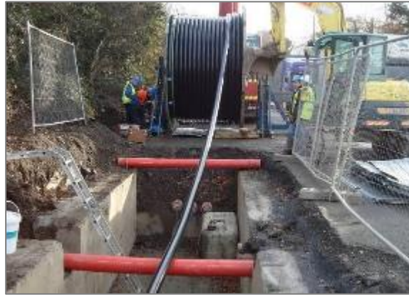
Figure 11 - HV cable pulling procedure (Typical drum set-up)
