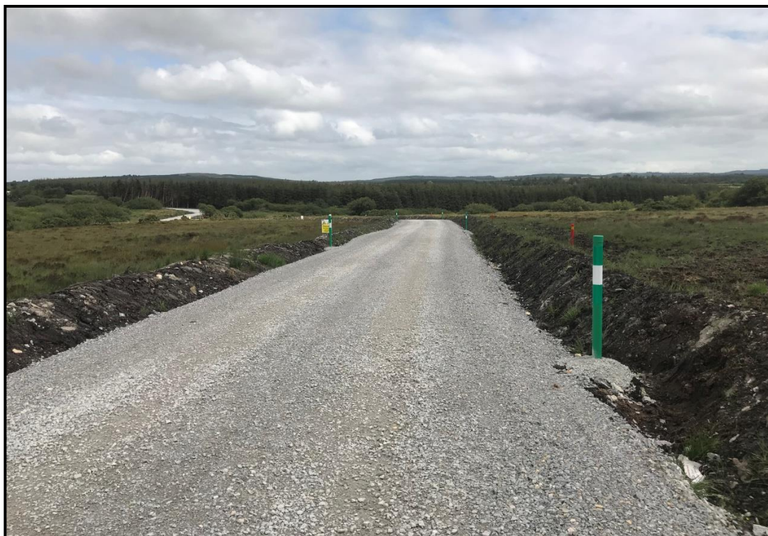
Figure 4.4 Typical floated road on a wind farm
