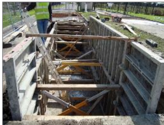
Figure 8 - Typical joint bay under construction (in-situ)
