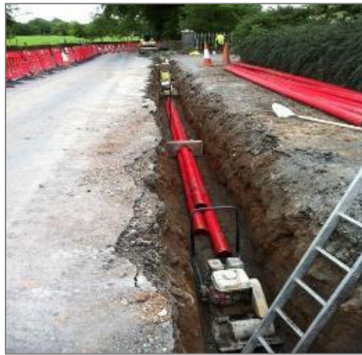
Figure 2 Typical 110kV Underground Duct Installation
