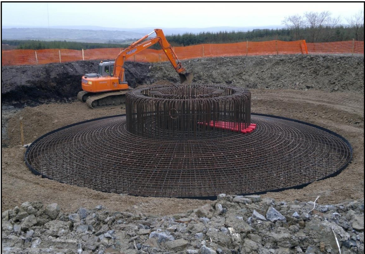
Figure 4.10 Typical construction of a wind turbine base
