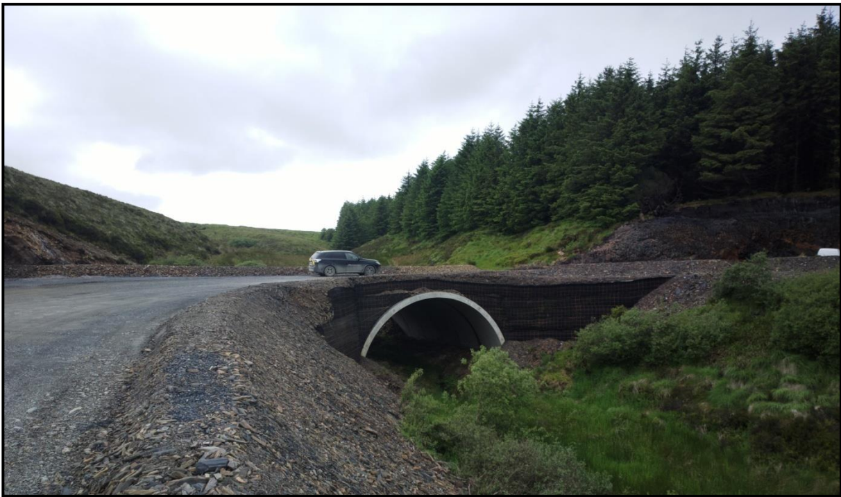
Figure 4.7 Completed clear span pre-cast concrete culvert crossing over existing watercourse
